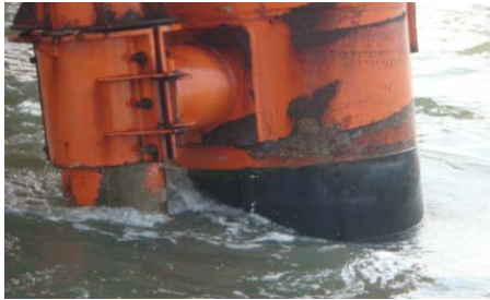
图 7 二个冰期后桩腿外观情况 Fig.7 The appearance of legs after two ice ages
