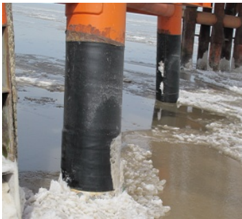
图 6 一个冰期后桩腿外观情况 Fig.6 Appearance of legs in a post glacial period
